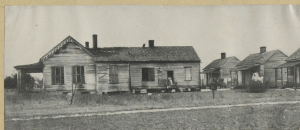
"BIG HOUSE" AND NEGRO QUARTERS (The house is no longer in use although the Negro quarters are)
